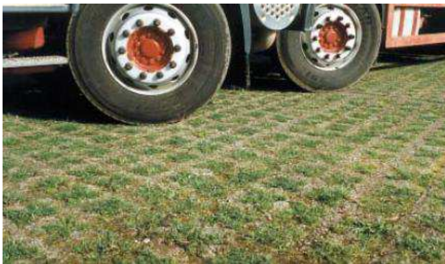
Figure 2-3 Concrete reinforced Grass Road
